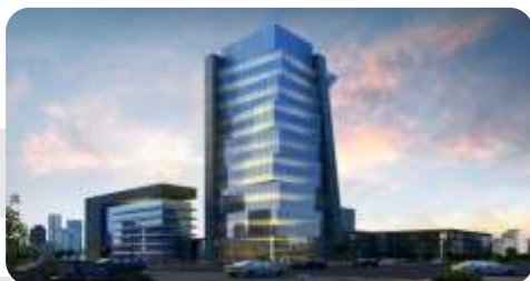
China Telecom Henan headquarters
