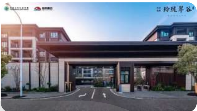
Nanjing CIFI Linglong Cuigu– Ever Sunshine will provide service after delivered
