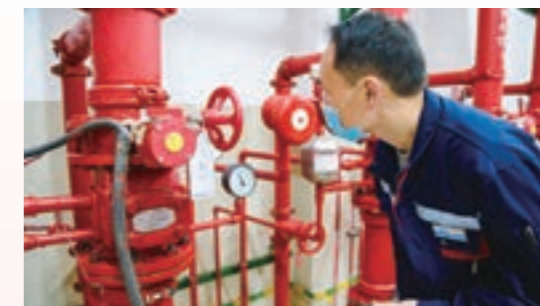
◆ Inspecting equipment rooms
