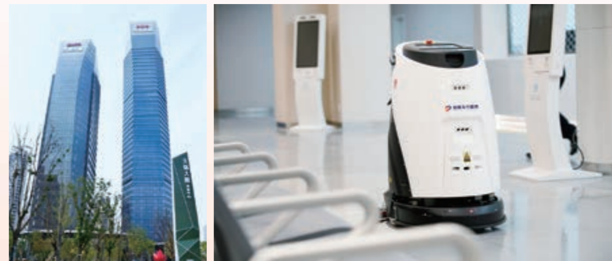
◆ Tiandu Building (天都大廈) is one of the landmark buildings in the CBD core area of Suzhou High-tech Zone. This project actively incorporates professional and smart service contents, such as Zeyue Commercial, interactive system of intelligent robot, AI camera, smart patrol, smart entrance guard and smart parking. It is a benchmark landing project serviced by Zeyue Commercial & Office under CIFI Ever Sunshine Services.
