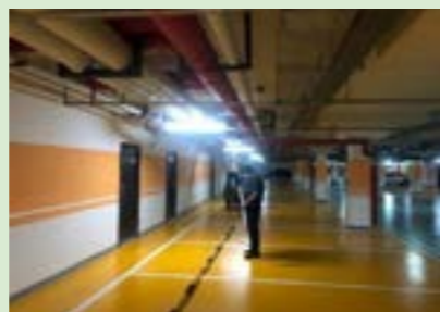
◆ Renovation of energy-saving lamps in the basement of Yinshengtai area
